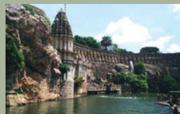
Fig. 4b. Chittorgarh Fort, Rajasthan
